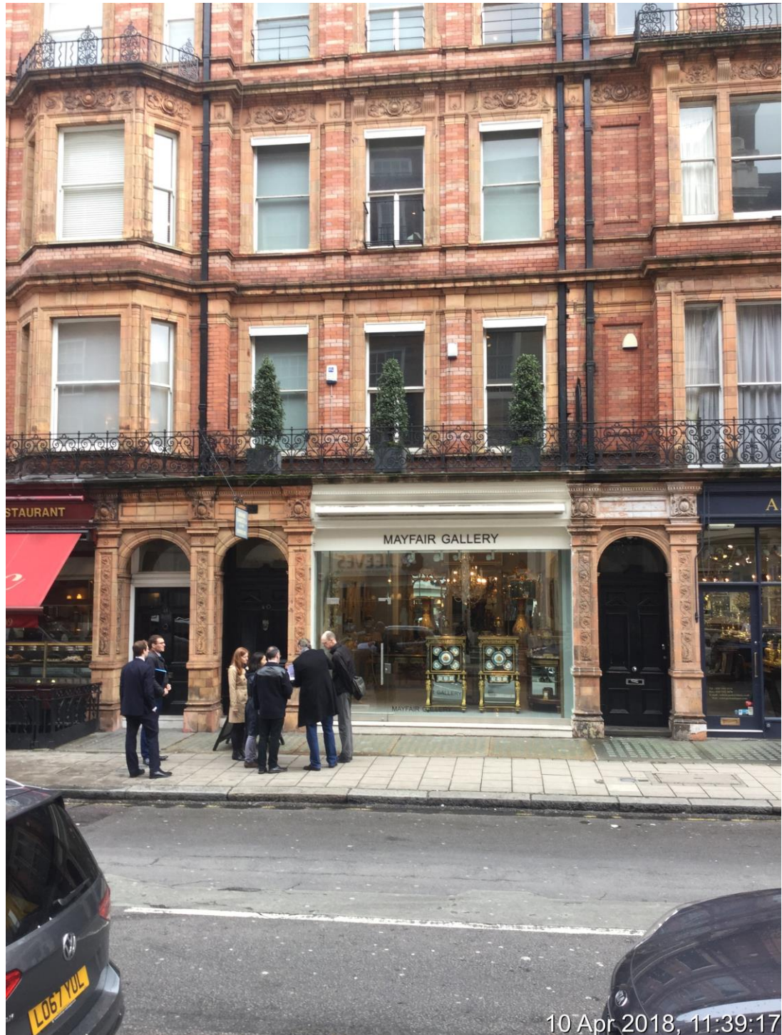
South Audley Street Frontage
