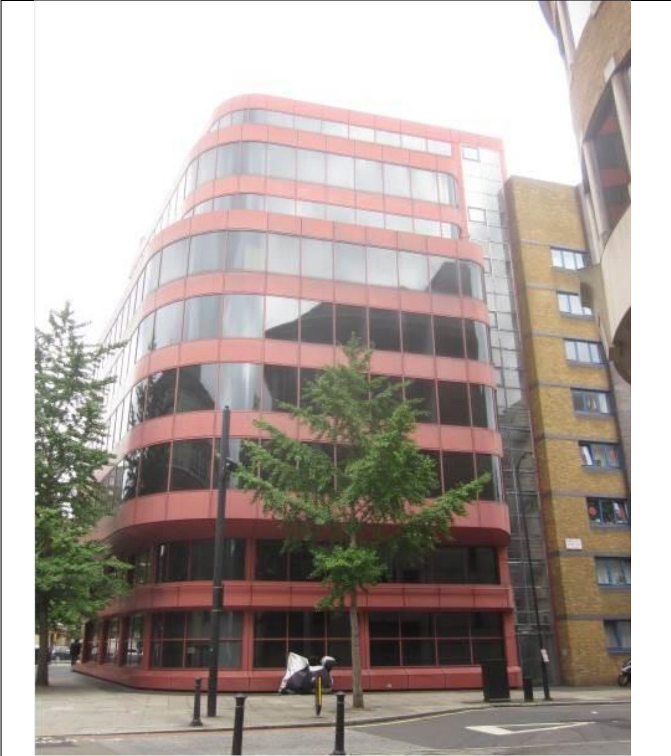
Application site as seen from Harcourt Street and Marylebone Road intersection.
