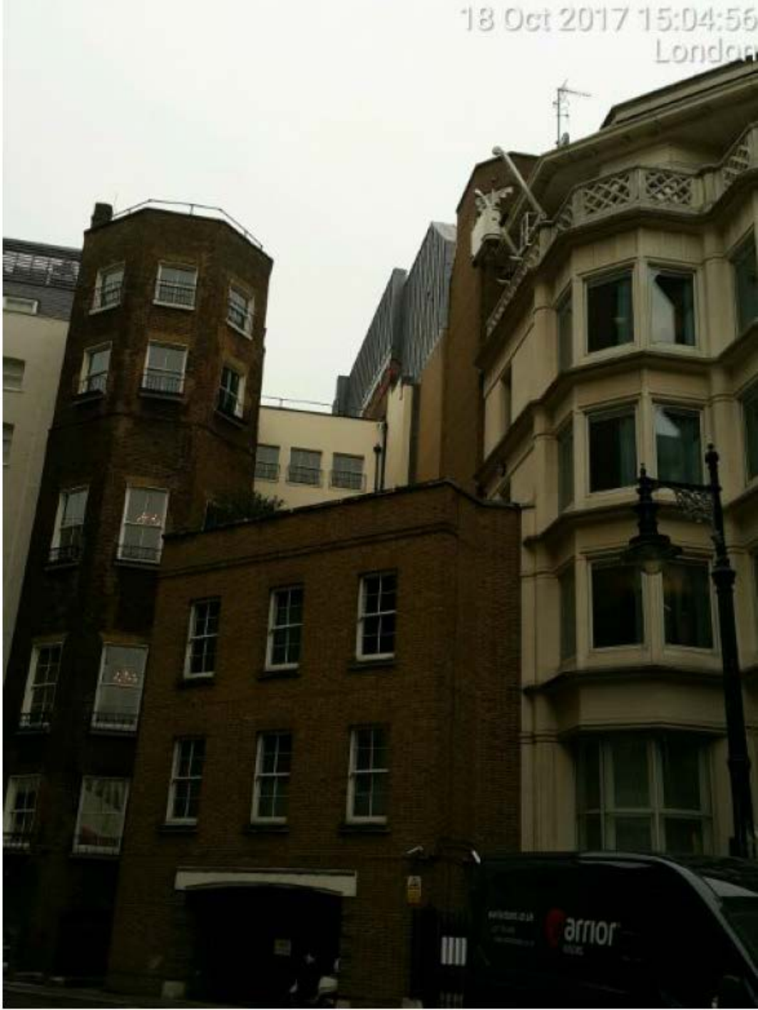
From junction of Bruton Lane and Berkeley Street / Berkeley Square looking north-east.
